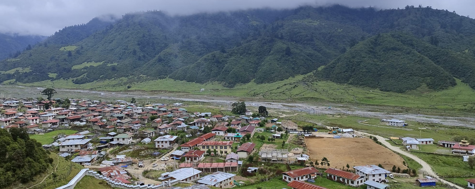
Sakteng village, upstream of the Gamri I Hydropower Project
